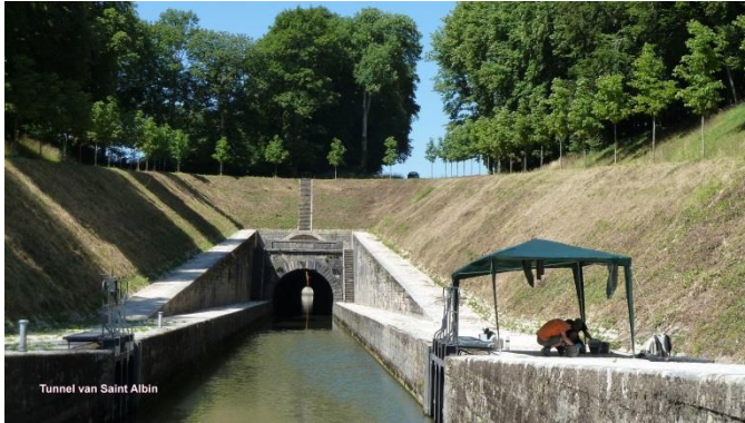
Tunnel Saint Albin
