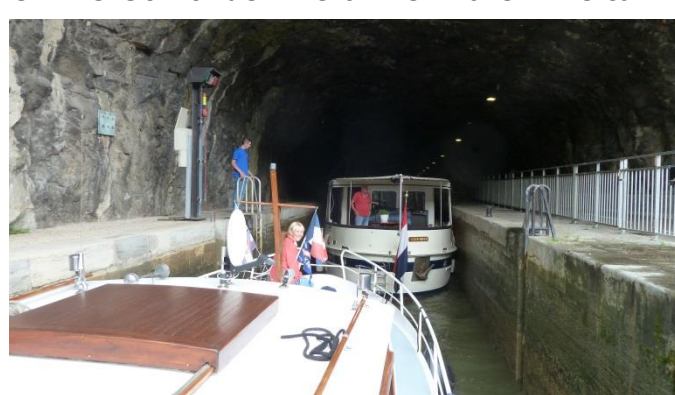
Sluis in tunnel
